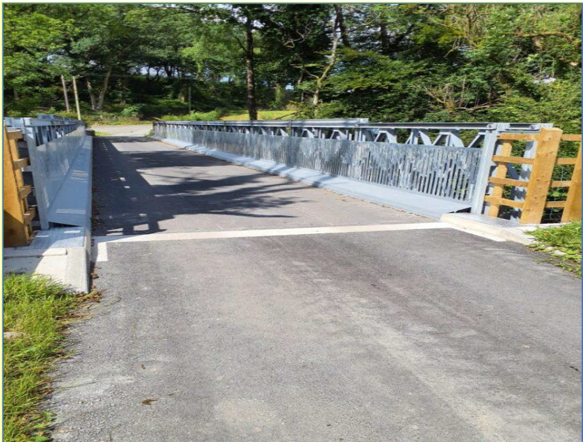
Glanrhyd Bridge replacement 2023
