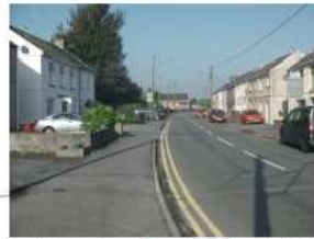
View of Ashburnham Road Looking West (No Neighbouring Properties)
